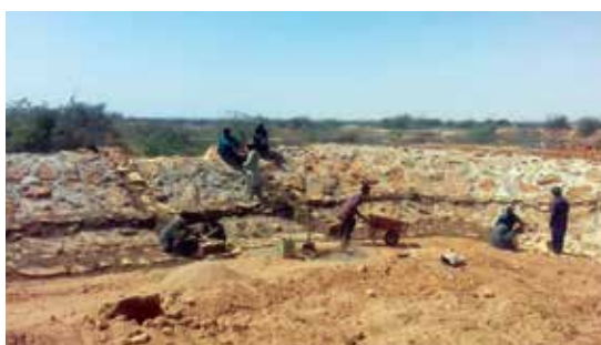
Construction of check dam in Kohistan.
