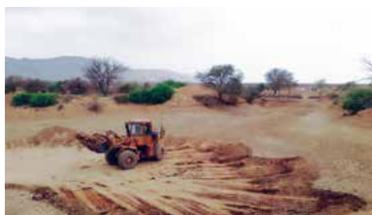
Initial construction view of check dam development.
